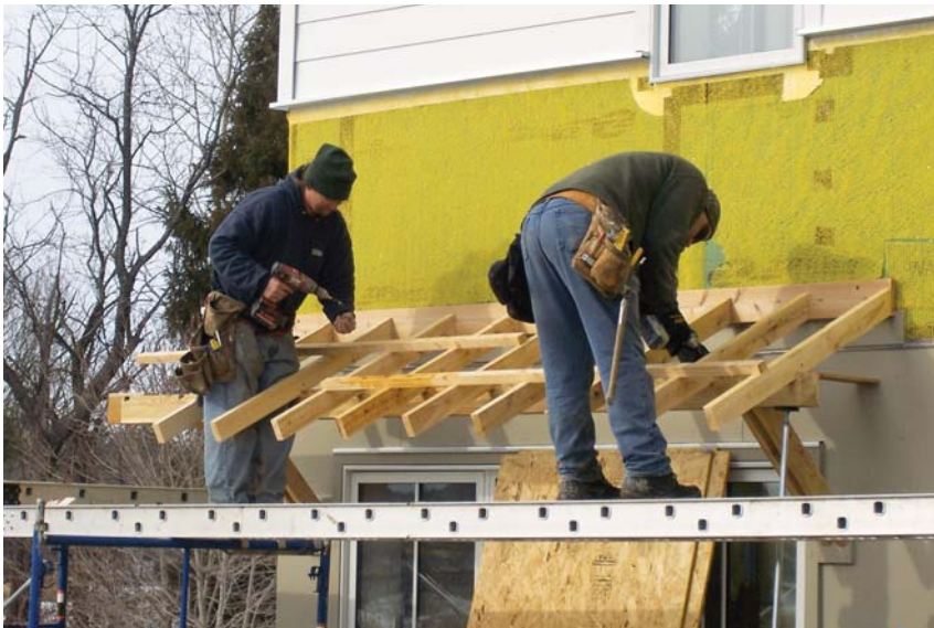
Figure 4. Fixed awnings shade south-facing windows from high summer sun while allowing lower-angled solar gain during the winter months.
