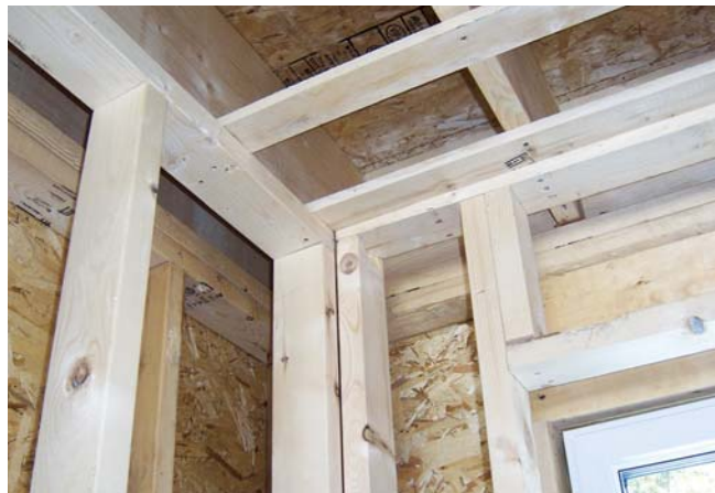
Figure 5. The bottom plates of the inside walls sit directly atop the slab's perimeter insulation, preventing a direct mechanical connection to the concrete. To hold the walls parallel to the exterior walls, the author used plywood standoffs and sealed beneath the plates with expanding foam (left). Single-stud corners reduce thermal bridging and allow fuller insulation coverage. Wall plates running parallel to the ceiling joists are nailed to 1x3 ceiling strapping, eliminating redundant framing (above).
