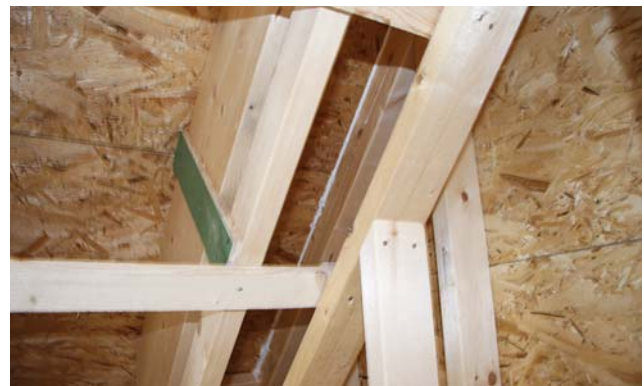
Figure 7. Ties made from Zip sheathing scraps connect 2x3 extensions to the 2x10 rafters to create a 14-inch-deep insulation cavity (left). Blocking between rafters is fully caulked around the edges to prevent air movement and moisture migration through the cellulose insulation (below left). Gable walls are framed with double top plates in lieu of end rafters, breaking conductivity through framing members and creating an unobstructed insulation cavity (below).
