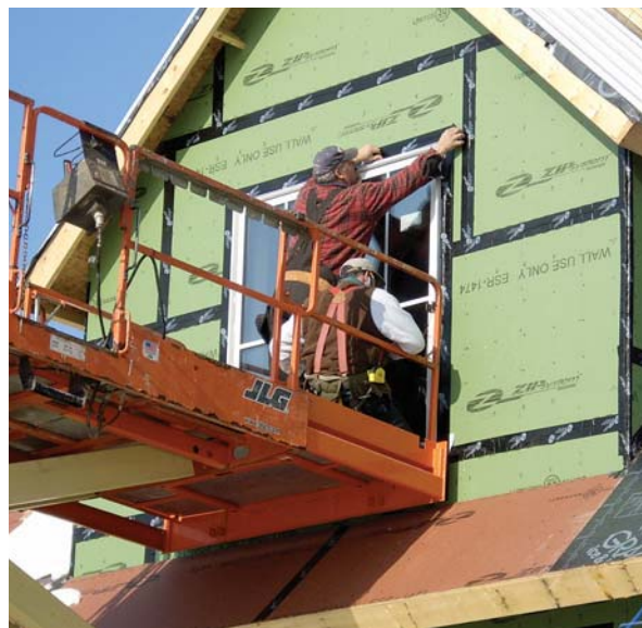
Figure 2. With the seams taped, Zip System sheathing provides a water-resistant air barrier under the siding.
