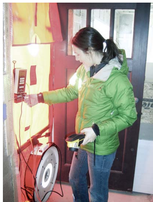
Figure 8. Blower-door testing at the weathertight stage is effective for early detection and treatment of air leaks in the envelope. The author achieved remarkable levels for this stage of construction.
