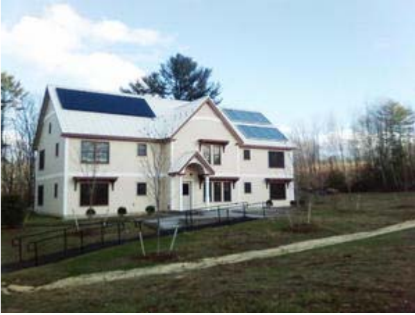
Vinton Hall's rooftop solar array is expected to generate half of the eight-unit building's power needs.
